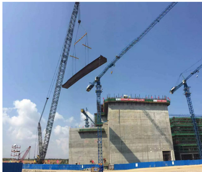
Figure 3.46: HTR-PM roofwork in September 2015
